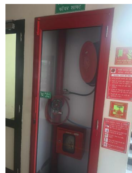
Fire hose reel and hydrant system.jpeg
